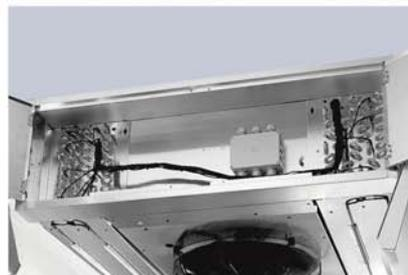
The **IDE** range of dual discharge unit coolers has been specifically designed for applications in large cold rooms and refrigerated storerooms with limited height, suitable for the preservation of fresh and frozen products.
